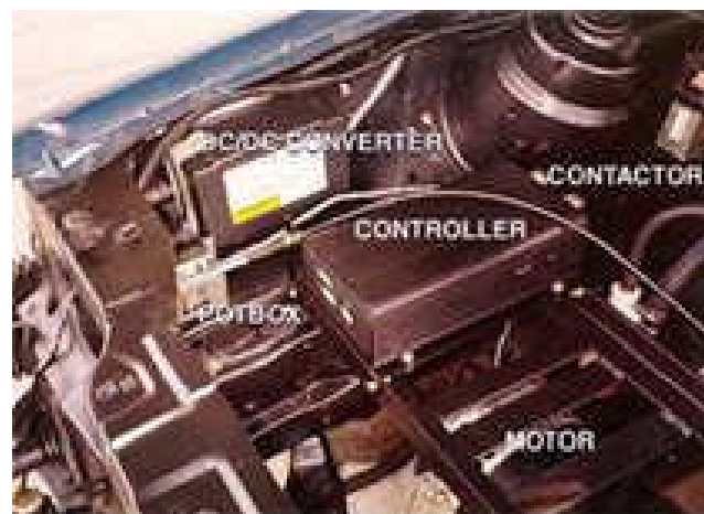
Electric components installed
